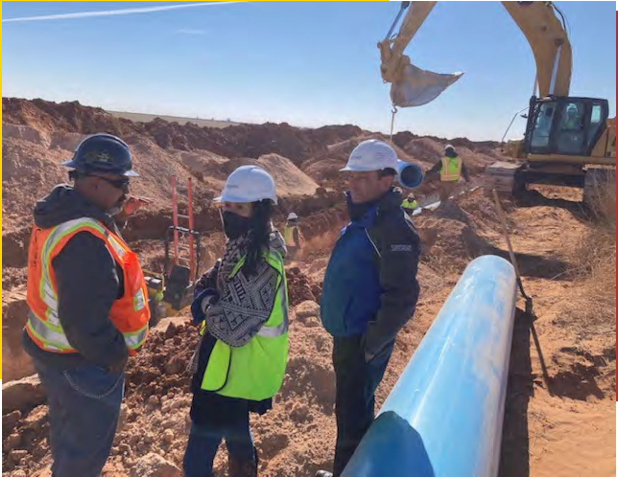
Congresswoman Leger Fernández at ENMWUA Pipeline construction site.
